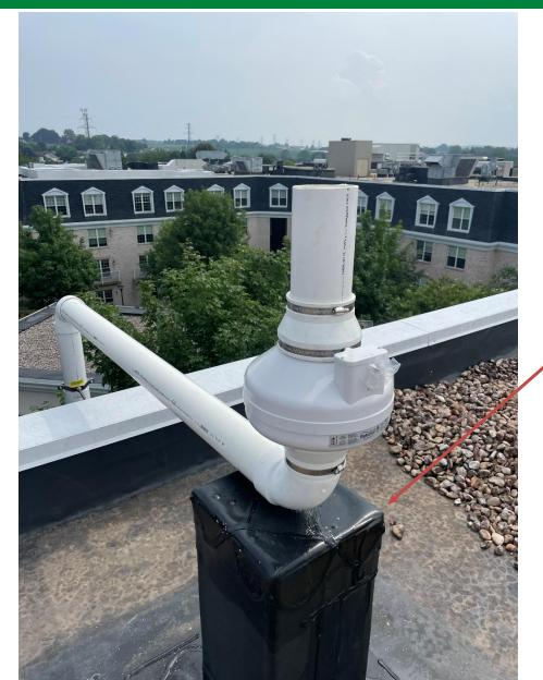
Box for fan support had to be installed by roofer.
