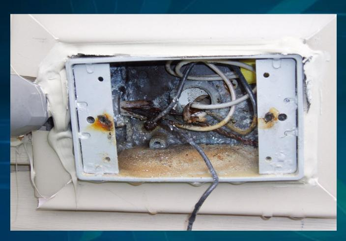
Completely rusted out, filled with water, if your drilling your own hole in the top use a Meyers hub
