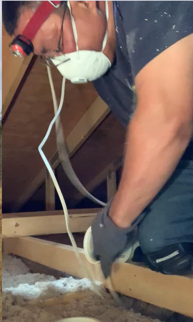
Johnny installing radon pipe in attic
