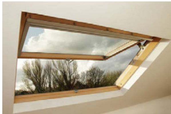
Skylight for natural daylighting. Photo: U.S. Department of Energy
