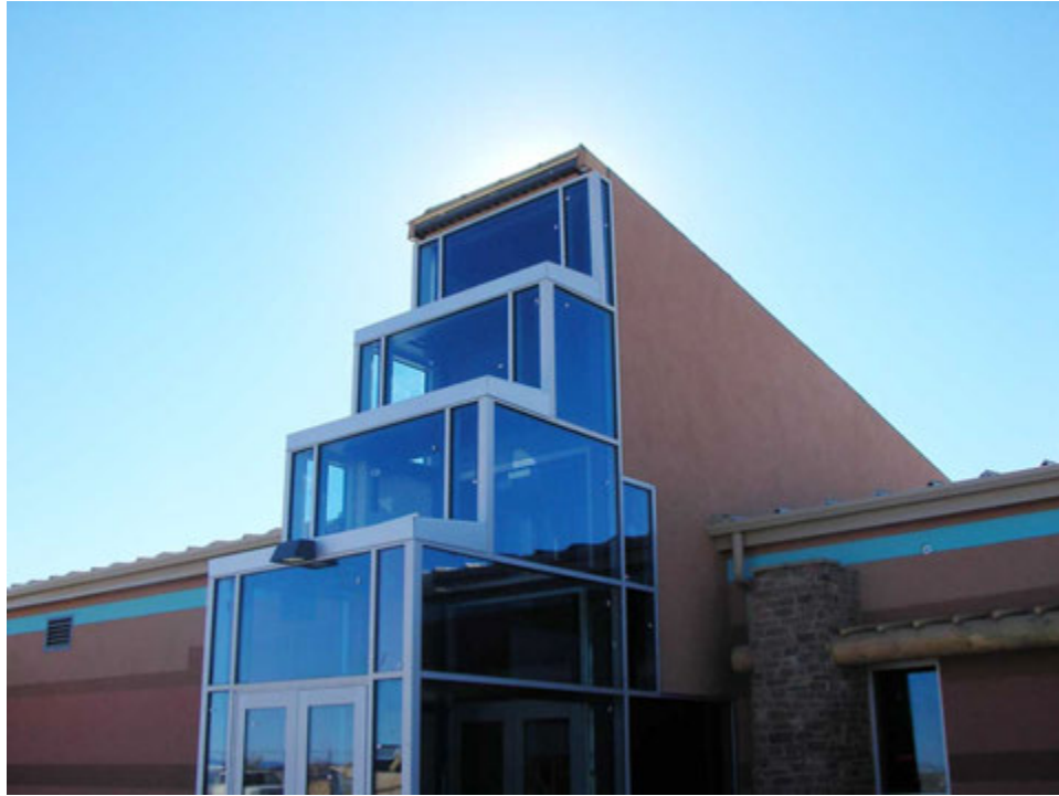
Kayenta Township, Navajo Nation, Arizona: Northeast Arizona Technical Institute for Vocational Education. Photo: Kayenta Township Building Department
