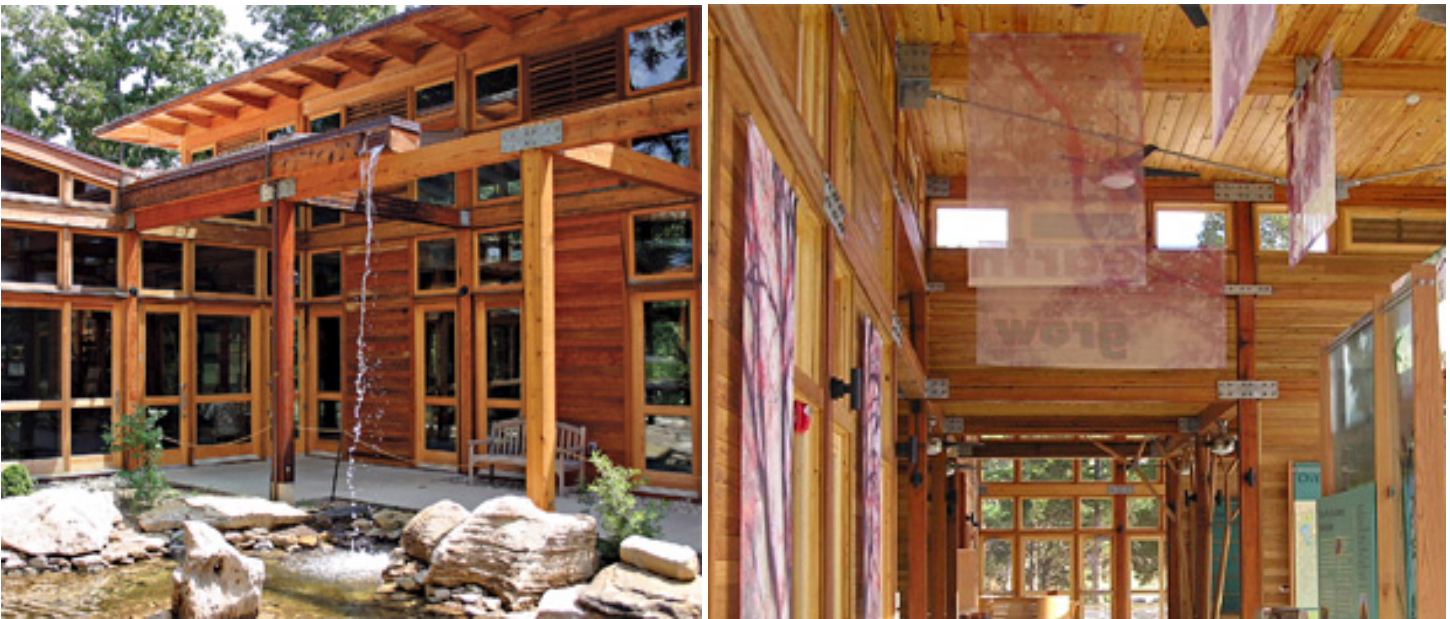
The Bernheim Arboretum Research and Visitors' Center used reclaimed materials, mechanical connections and reconfigurable modules to reduce waste and greenhouse gas emissions. Photo: Lifecycle Building Challenge via William McDonough + Partners
