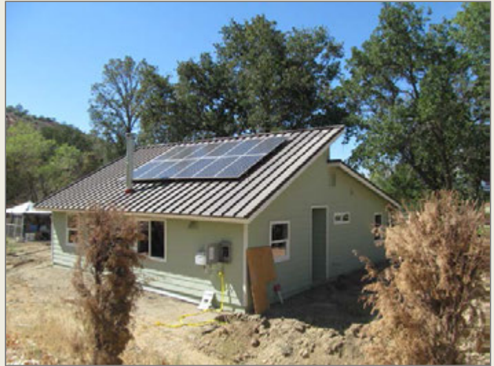
Big Sandy Rancheria home with solar panels. Photo: Jaime Collins
