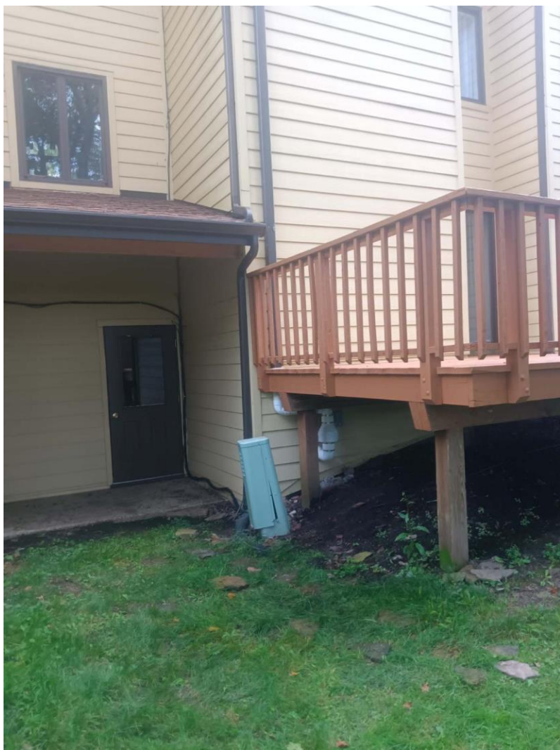
Actual Installation of fan at Butch's
